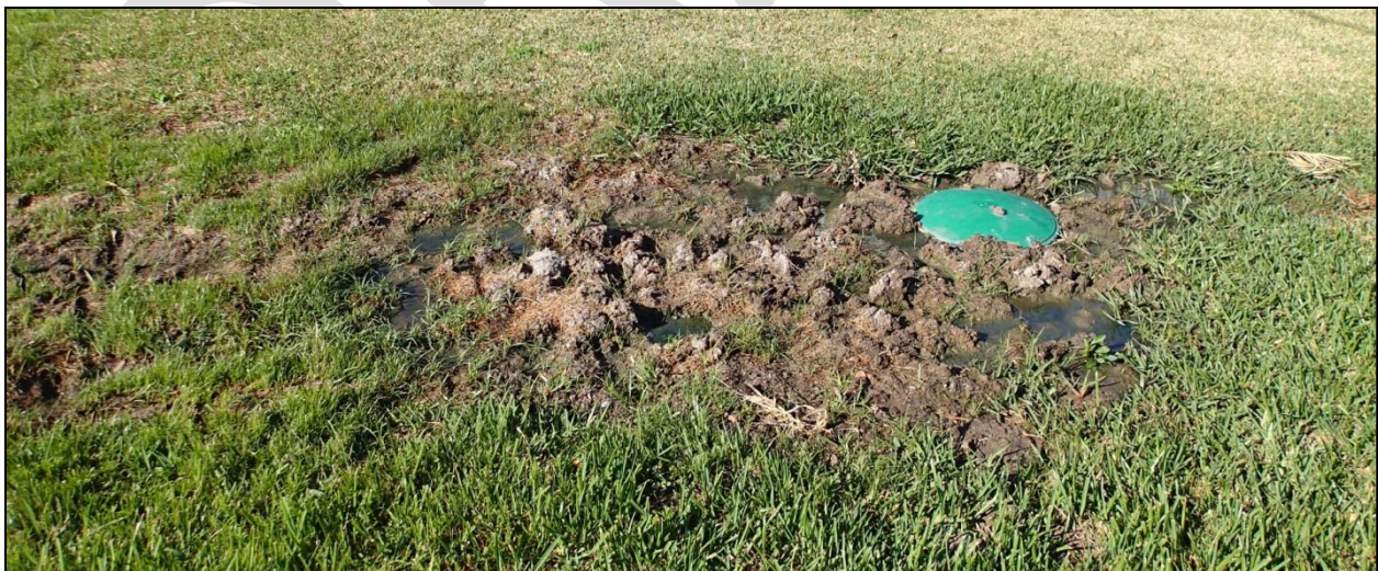
Figure 5.4. Surfacing effluent is a symptom of septic system failure that can be caused by several factors such as poor soil suitability, age of the system, or overloading. Photo courtesy of Ryan Gerlich.
